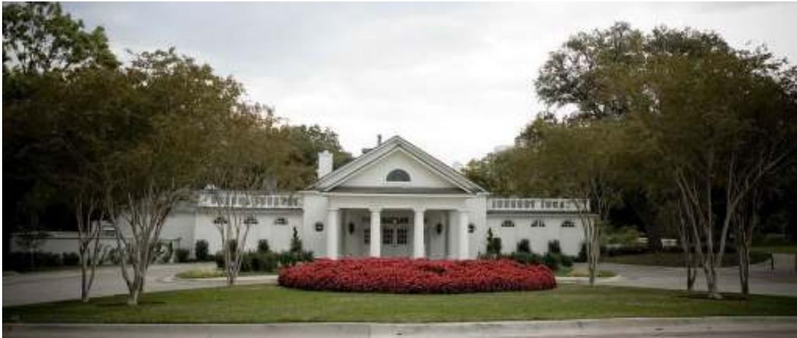
Arlington Hall at Lee Park ( Easterly View ) 3333 Turtle Creek Blvd. Dallas, Texas.
